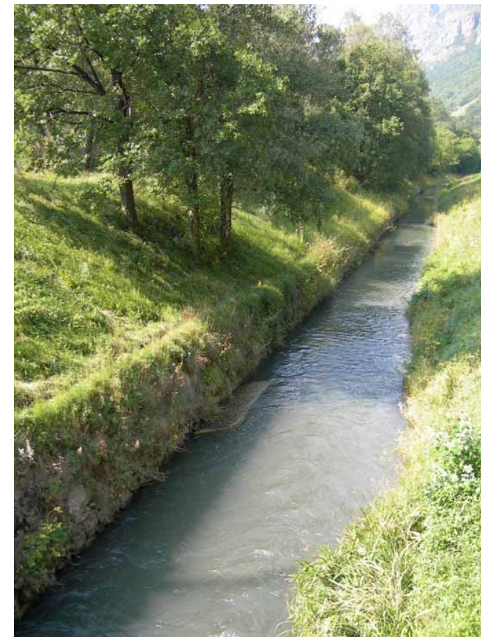
Open ditch with gravity driven flow
